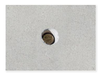
**Step 1**Penny-sized holes are drilled in the concrete slab
