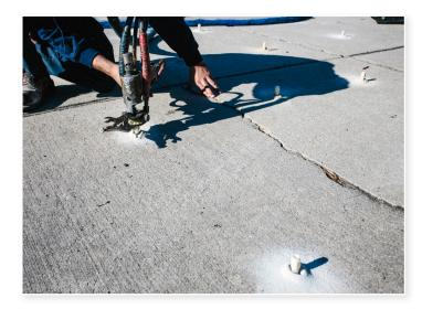
**Step 3**Expansive polyurethane foam is injected to support and lift the slab
