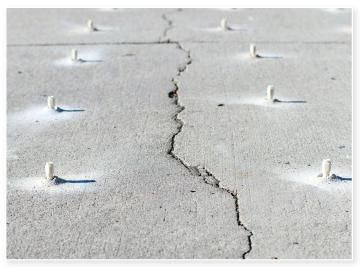
**Step 2**Temporary injection ports are installed
