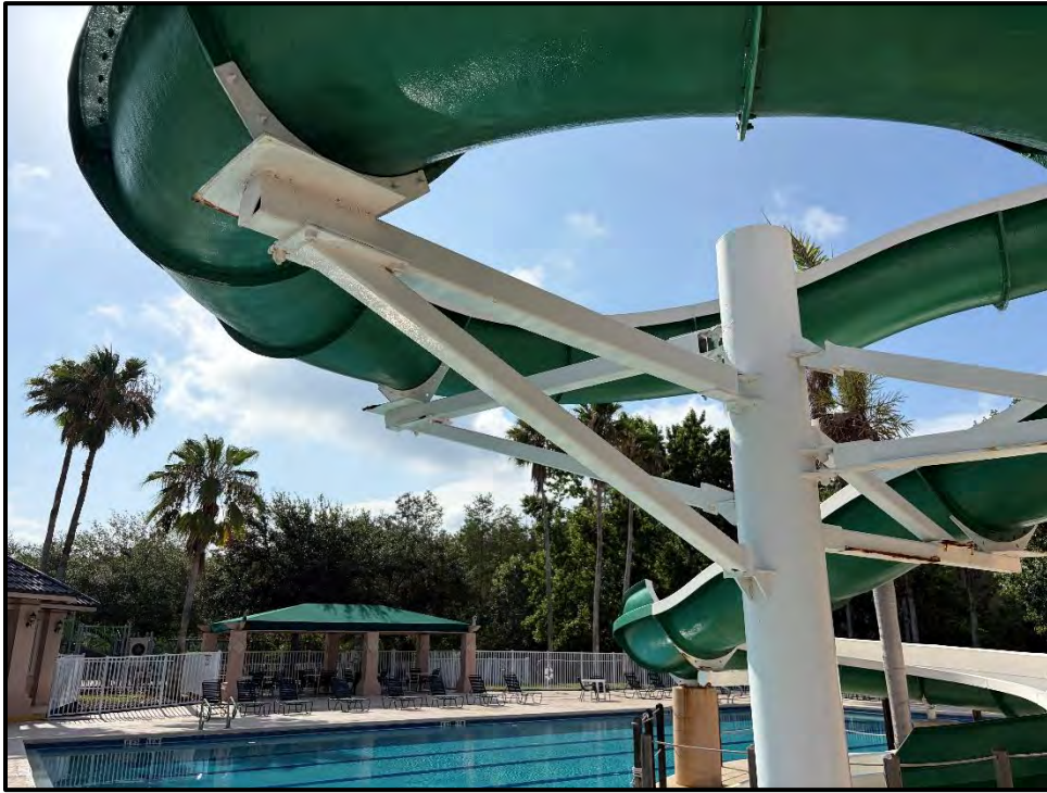
Photo 43– Support PKT-8 overview.
