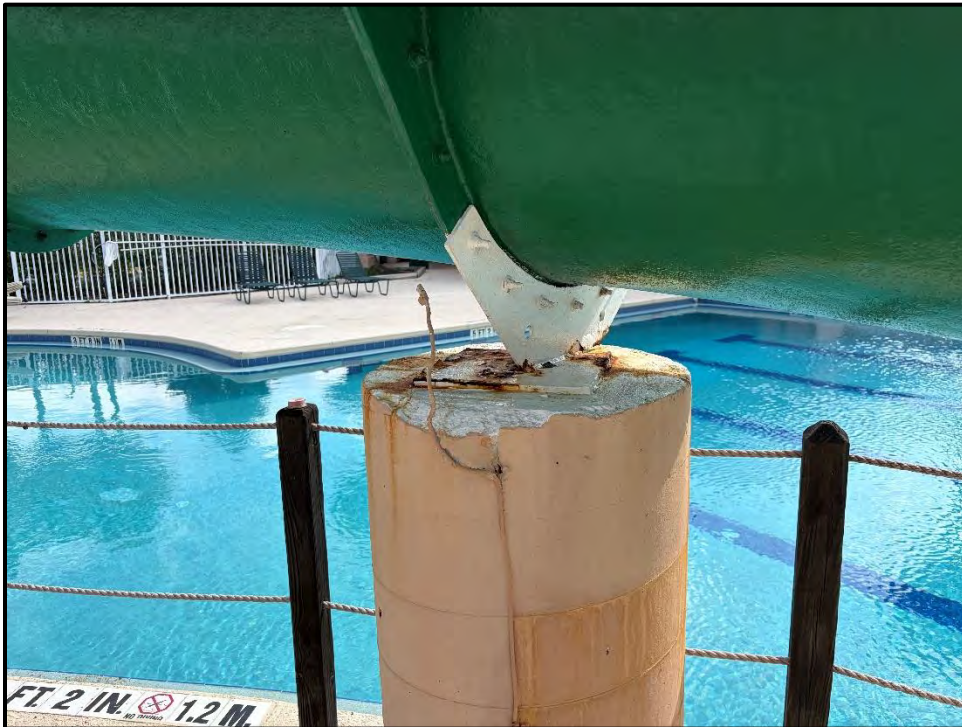
Photo 14 – Support S-4 Overview
