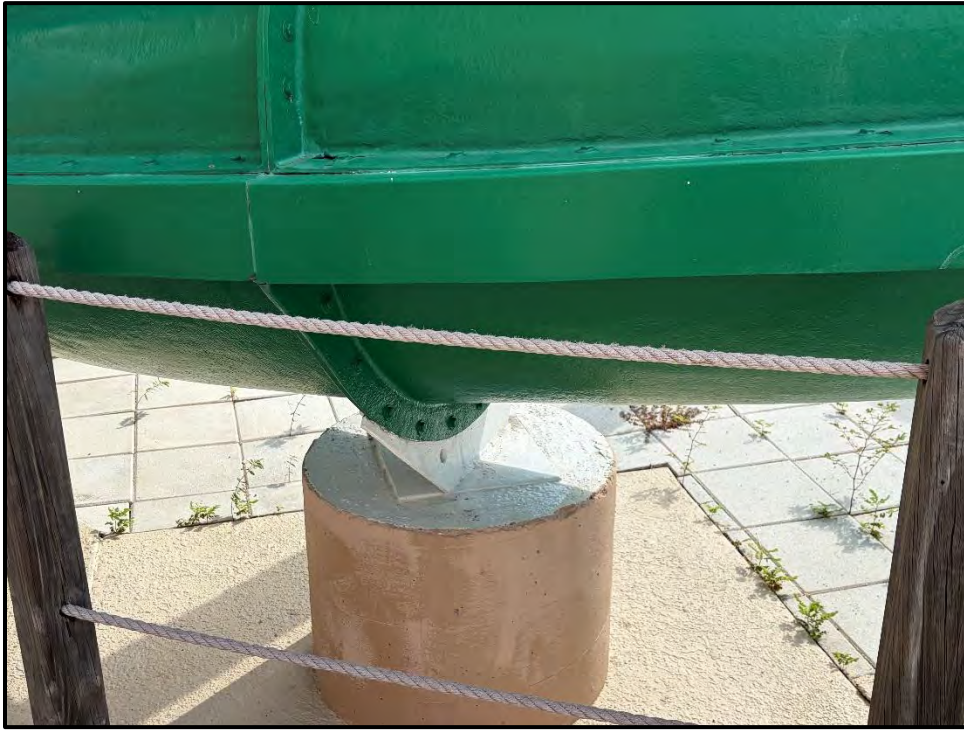
Photo 5 – Support S-2 Overview
