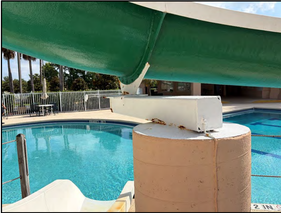
Photo 19 – Support S-5 Overview
