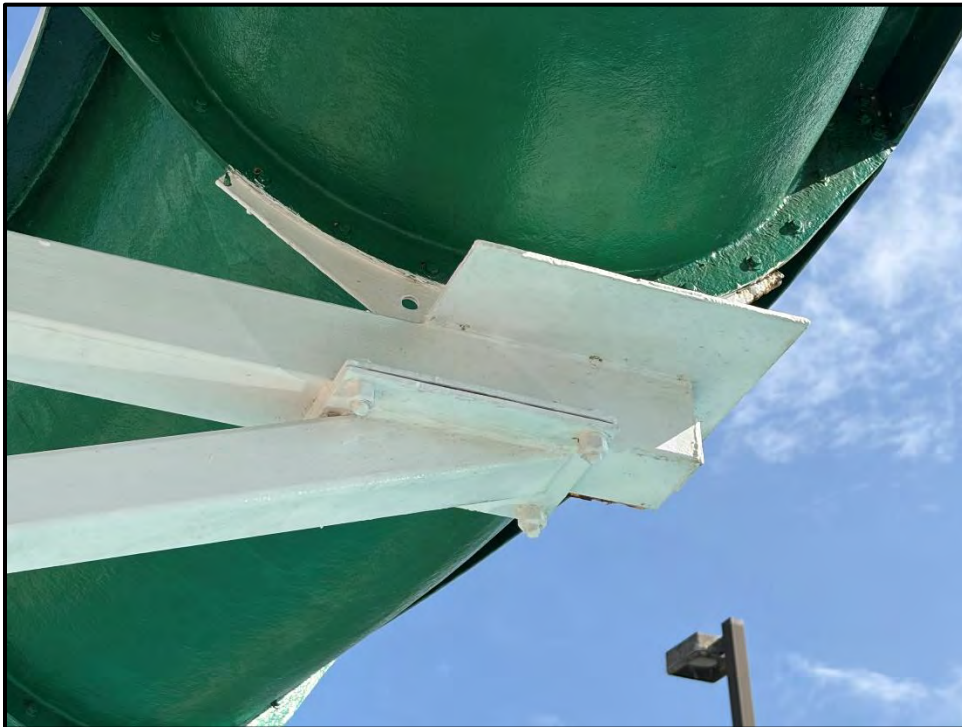
Photo 46 – Support PKT-9 overview.
