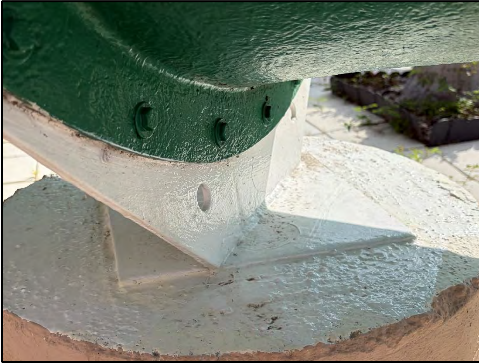
Photo 7 – Support S-2 in good condition
