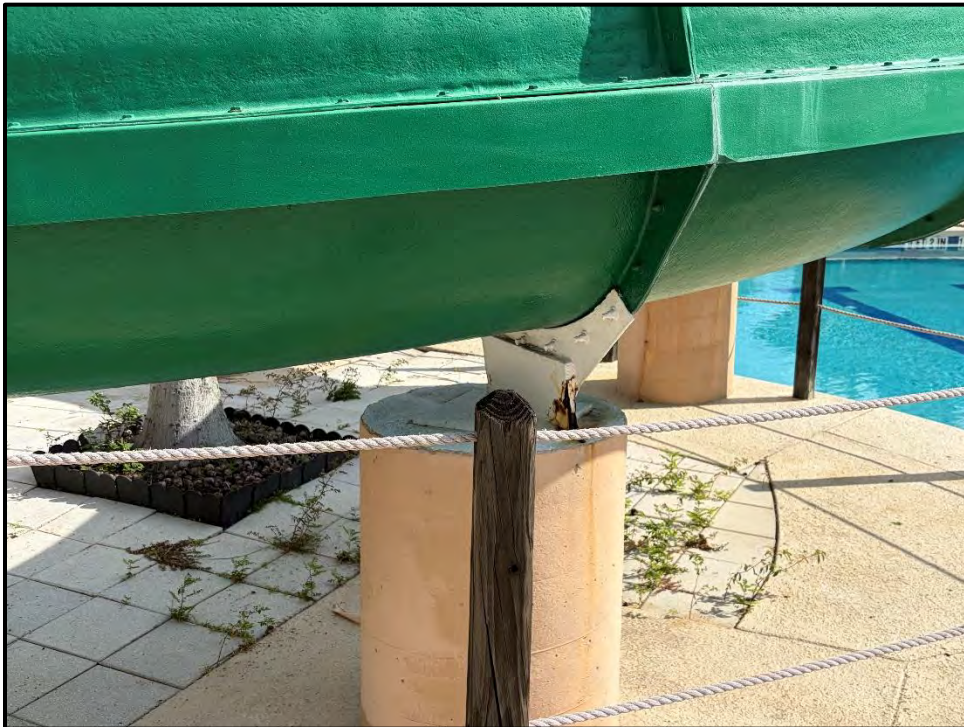
Photo 8 – Support S-3 Overview
