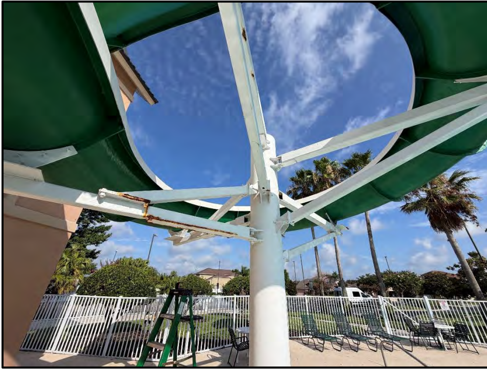
Photo 49 – Support column overview.
