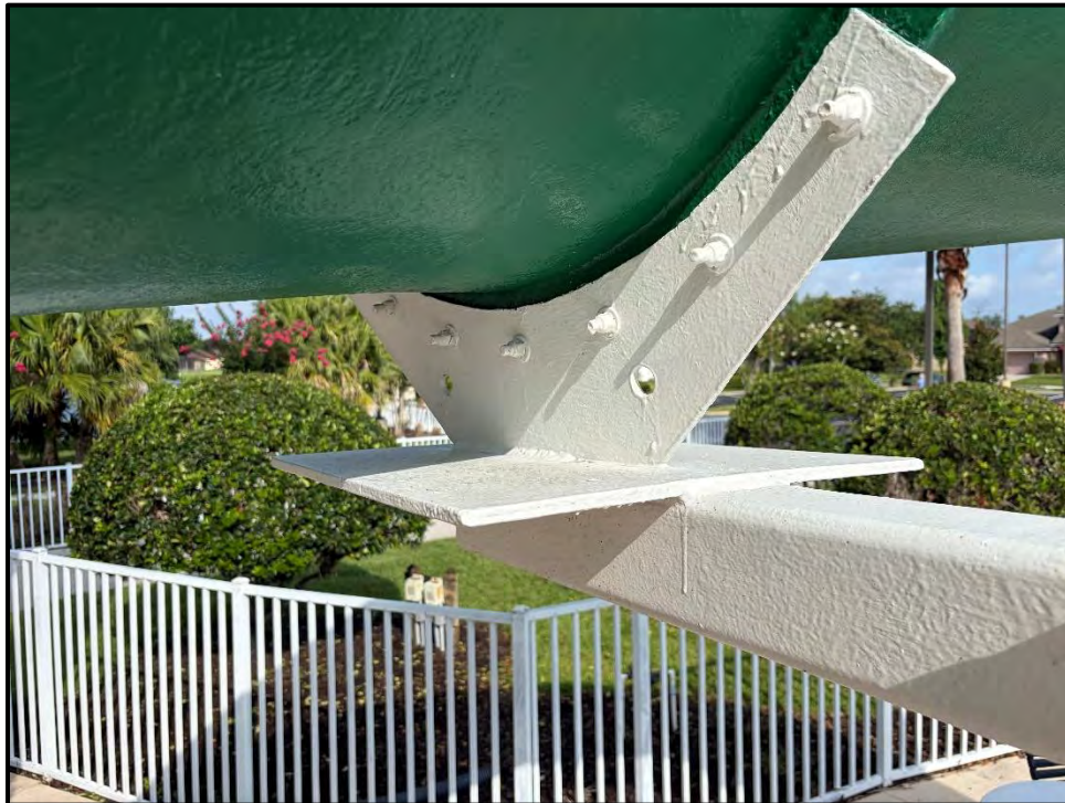
Photo 42 – Support PKT-7 yoke plate in good condition.
