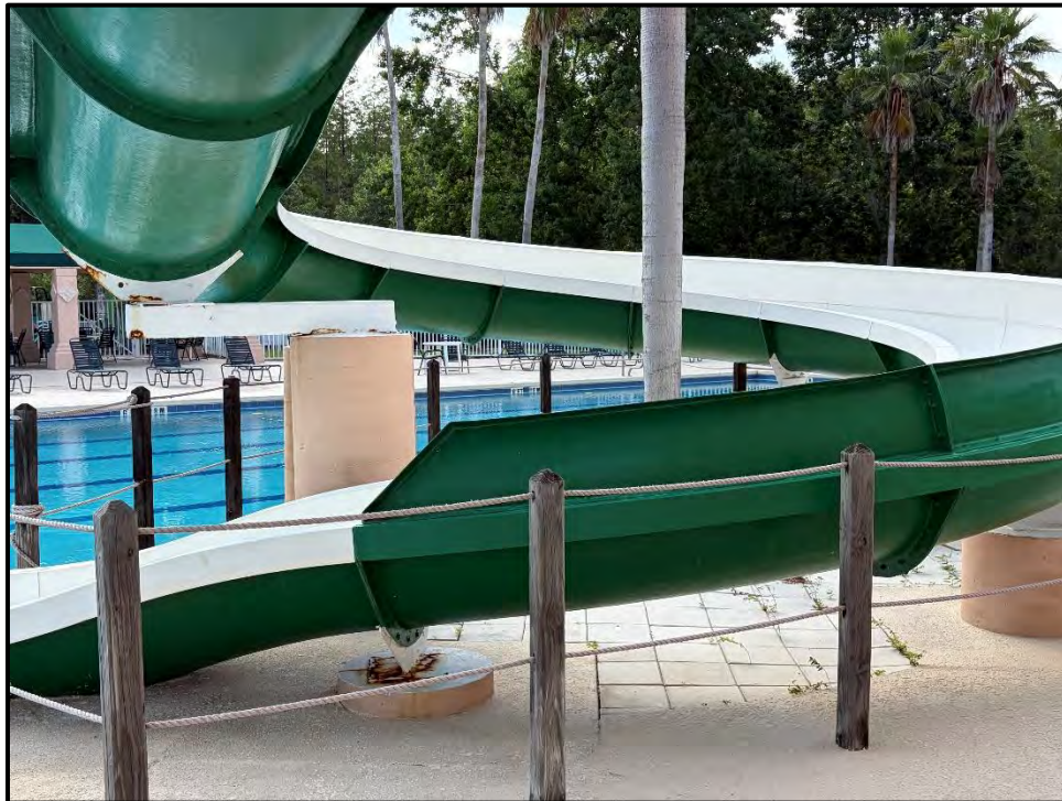
Photo 2 – Support S-1 Overview
