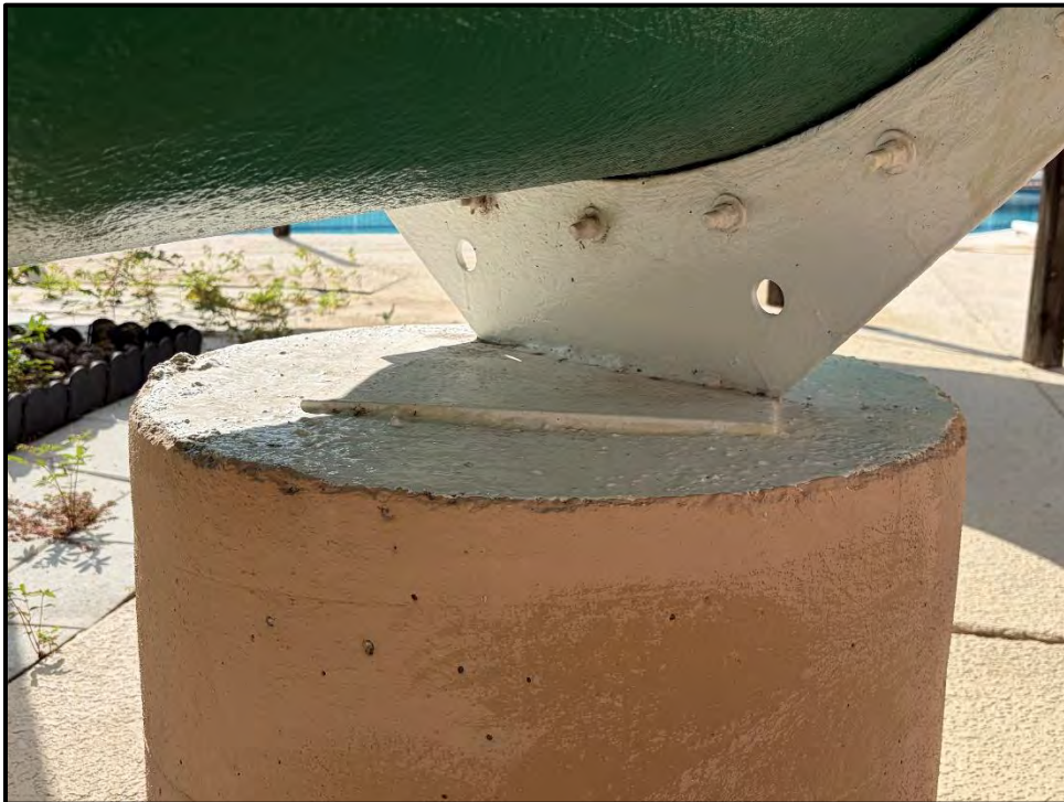
Photo 6 – Support S-2 in good condition
