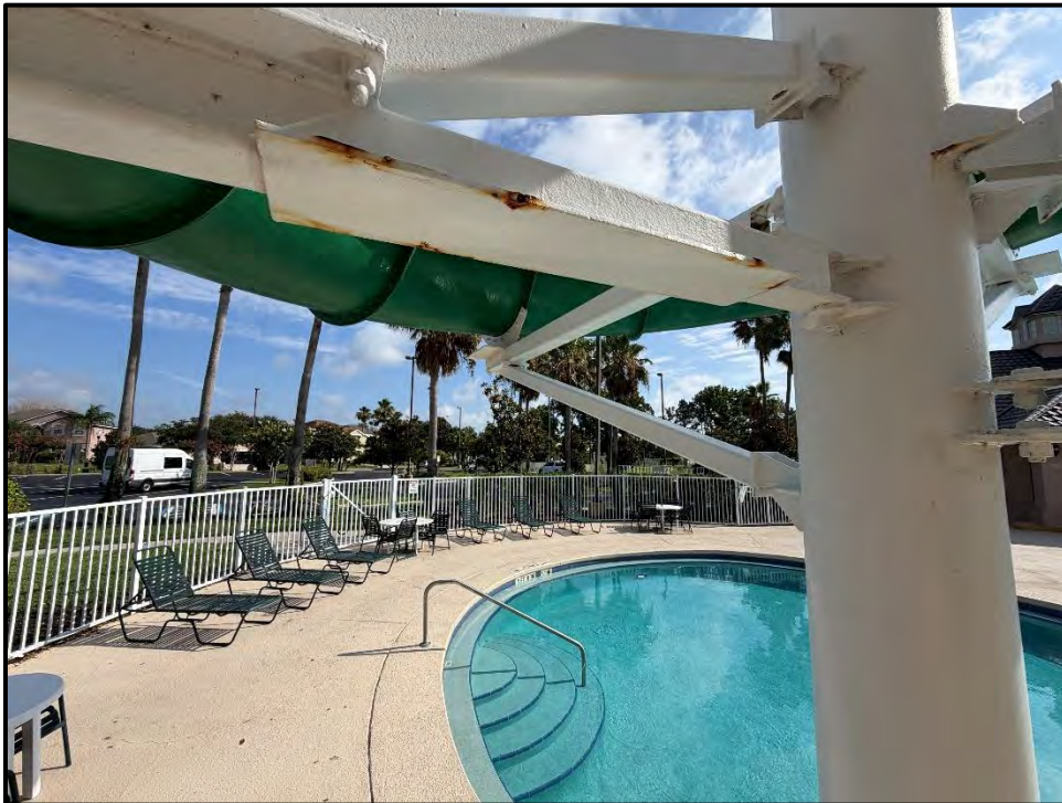
Photo 40 – Support PKT-7 overview.
