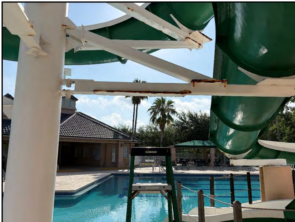
Photo 26 – Support PKT-6 overview.
